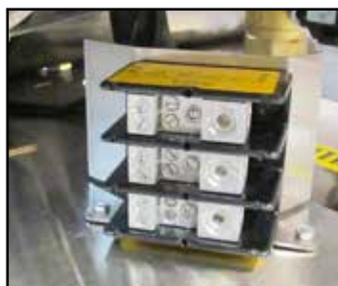
Fig. 3 - Booster terminal block
