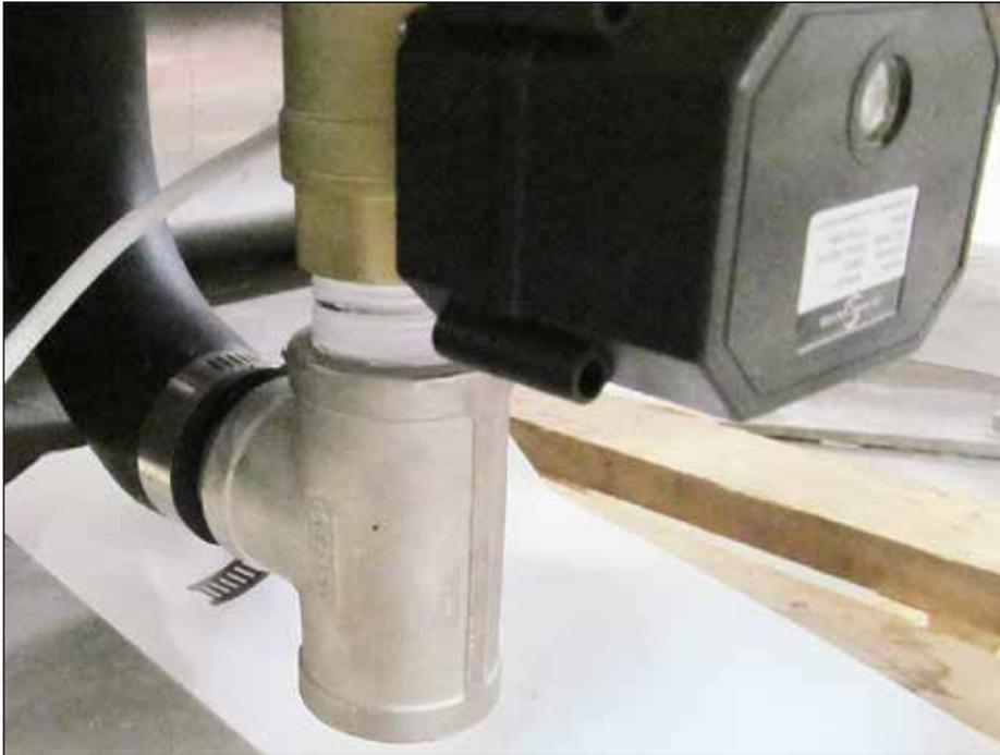
Fig. 7 - 1" NPT electric drain valve connection
