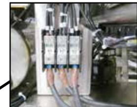
Fig. 10 - Power terminal block
