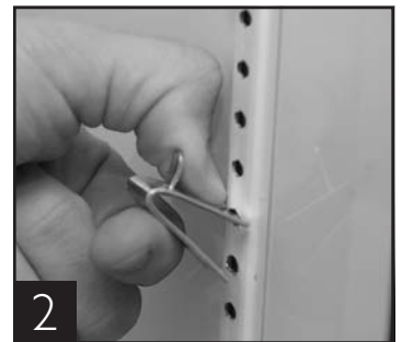
Installing bottom of the shelf clip
